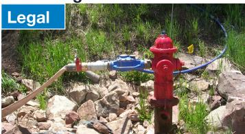
Proper way to hook up to a fire hydrant. Metered Hydrant - Hook Up
